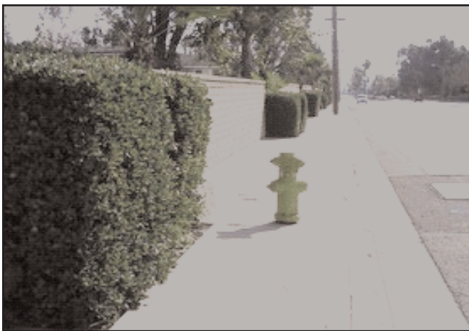
Path blocked by a fire hydrant in the middle of the sidewalk
